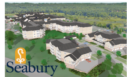
The new apartment homes
